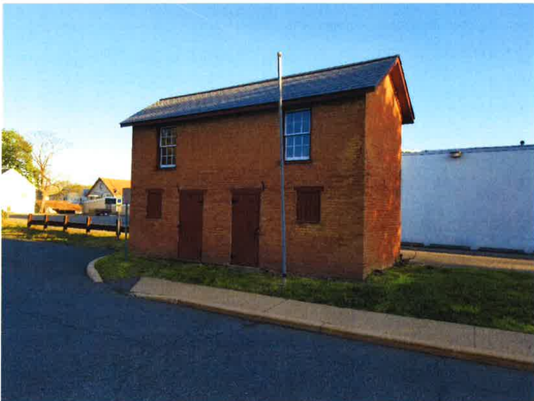
Small Brick Shed Building Looking Northwest
