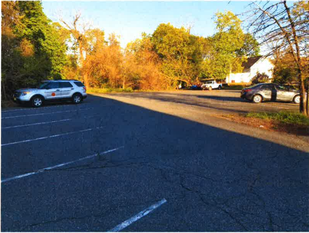
Rear Site View Looking West
